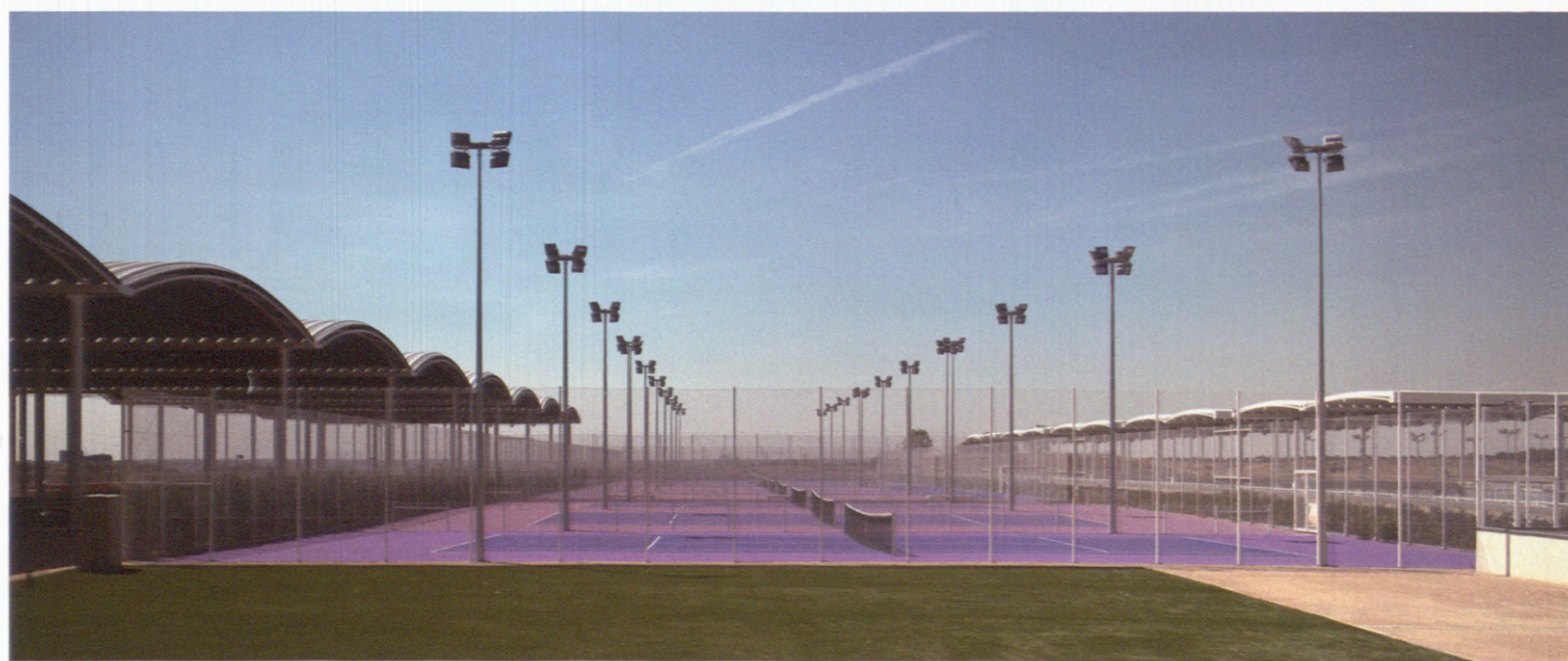
Pistas cubiertas de chapa plegada. Indoor courts covered by ribbed metal sheets.
